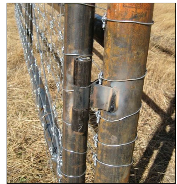
5 HINGE DETAIL NO SCALE
