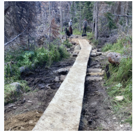
The finished Spruce Lake Trail bridge
