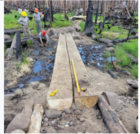
The new and improved Green Mountain Trail bridge
