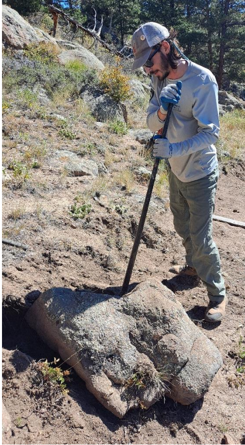
Nathan uses a rock bar to maneuver a boulder.
