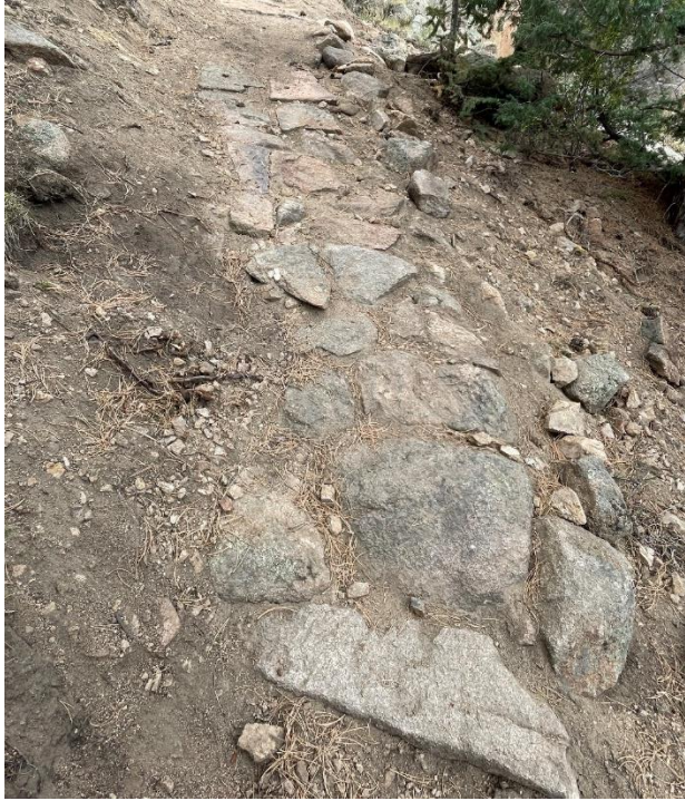
“Armoring” on switchbacks completed by Boulder Climbing Community’s Front Range Climbing Stewards.
