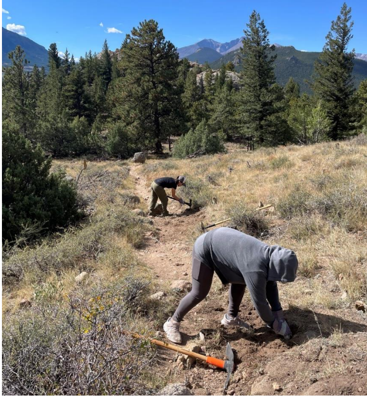
Maddie and Dalila use pick mattocks to remove rocks, shrubs, and widen the trail corridor.
