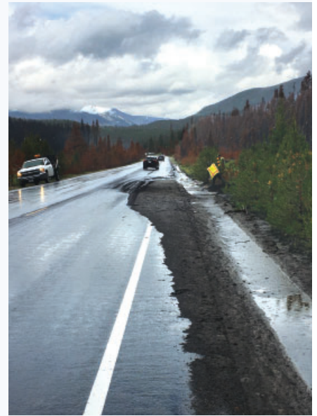
This summer's wet conditions may be helping vegetation rebound after the fire, but heavy rains also have caused some flooding, erosion, and sediment deposition. Here is debris along Trail Ridge Road on the west side of the park.
