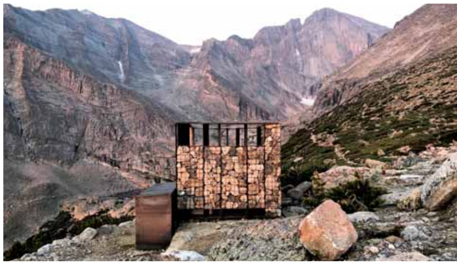
Sideview of completed Chasm Junction toilets in context
