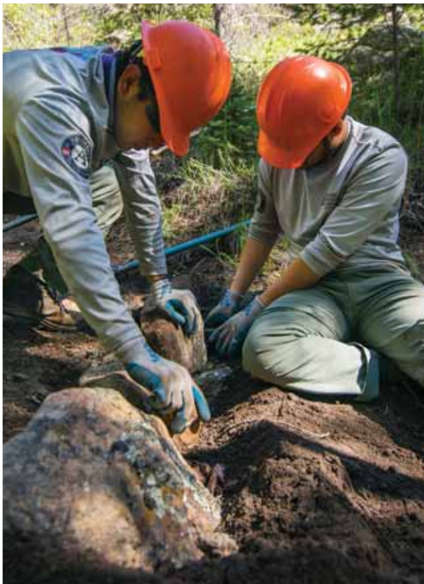
Conservation Corps Boulder crew members repair a trail by creating a rock check step.
