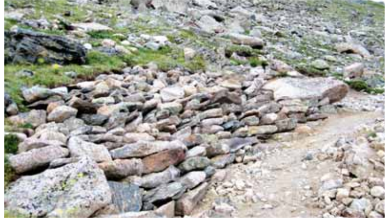
New rock wall supporting the tundra and preventing erosion on the Longs Peak Trail
