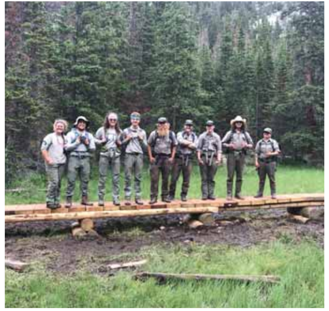
Estes Crew with NPS staff at the new bridge constructed this summer near Jewel Lake.
