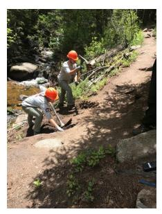
As warm weather melted snow in the high country, the Boulder Crew followed the snow line. On the South Boulder Creek Trail in the James Peak Wilderness, the crew helped to finish up a turnpike project and constructed waterbars, drains, and stairs to fortify a wet section of trail and protect surrounding riparian areas.
