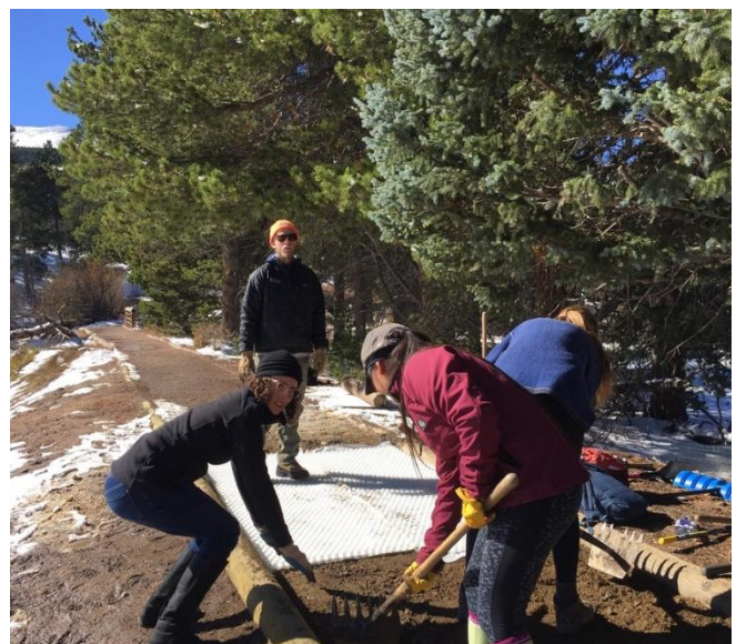
Volunteers fortifying the accessible Sprague Lake Trail with logs and erosion matting to prevent soil loss
