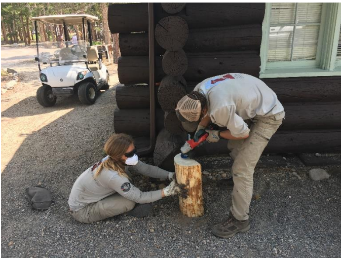
Moraine Crew works to restore the historic Ranger Station at Glacier Basin Campground by replacing a log footer.
