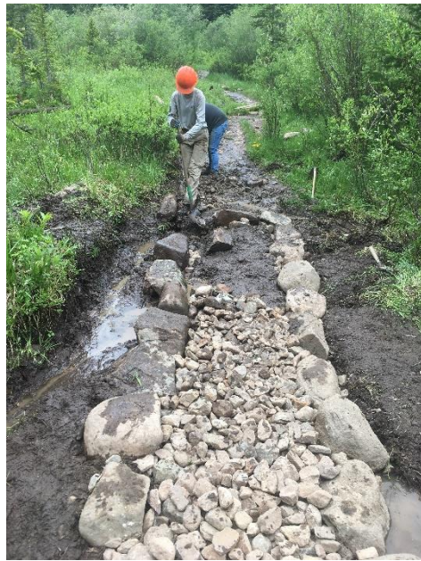
Boulder Crew constructs a turnpike on the South Boulder Creek Trail in the James Peak Wilderness.
