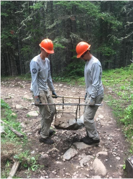
Boulder Crew constructs a turnpike on the South Boulder Creek Trail in the James Peak Wilderness.
