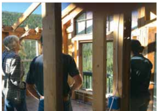
Wild Basin structure during the deconstruction (Photo: Carolyn Kilgore)
