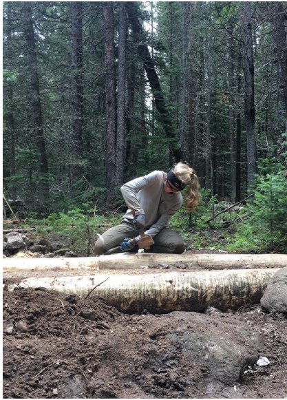
Photo: The crew working to set logs while replacing the turnpike at Bierstadt Lake.
