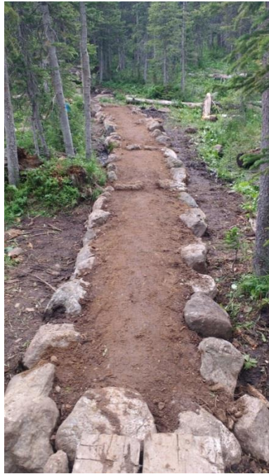
Photos: Completed turnpike on Diamond Lake Trail and check steps on South Boulder Creek Trail.
