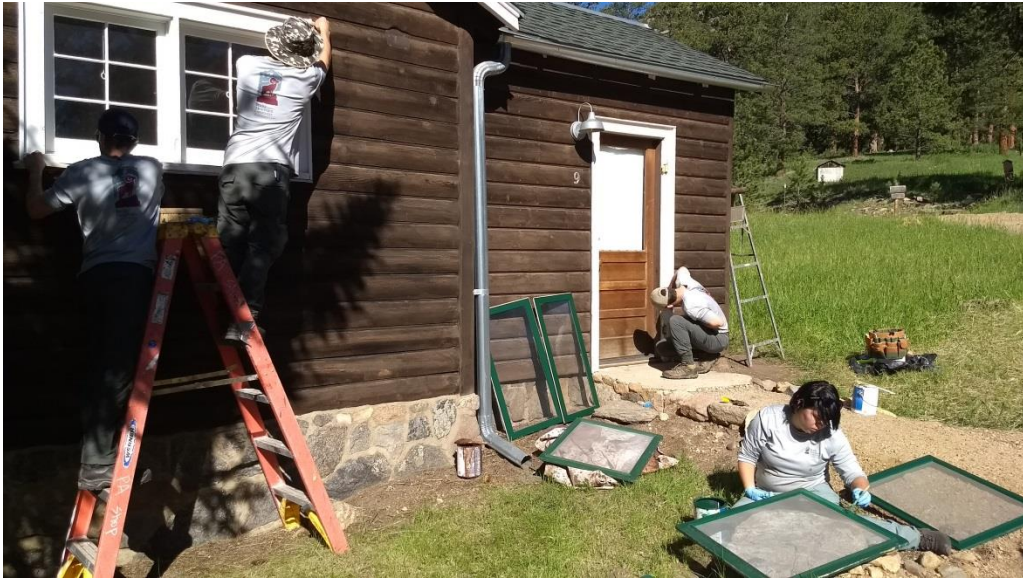
Photo: Crew refinishing the exterior of McGraw Ranch cabins.
