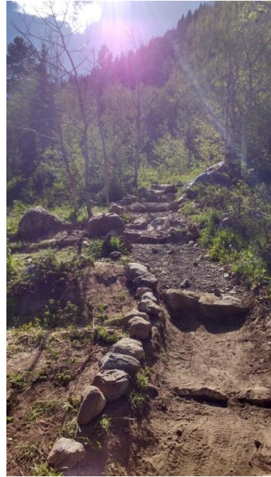
Photos: Completed turnpike on Diamond Lake Trail and check steps on South Boulder Creek Trail.
