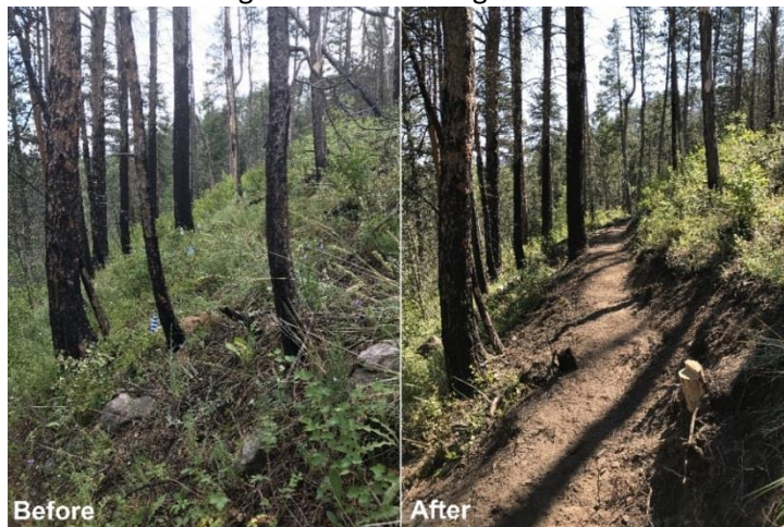
Photo: Before and After of the crews digging new tread for the Young Gulch Trail.
