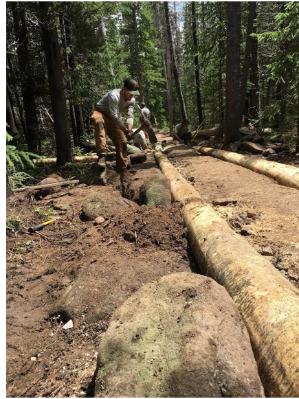
Photo: The crew working to set logs while replacing the turnpike at Bierstadt Lake.
