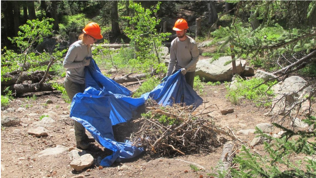
Photo: Crew decommissioning social trails with “duff,” loose sticks, pine needles, and debris.
