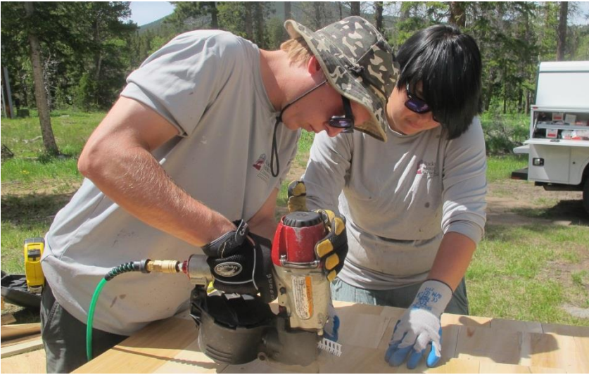
Photo: Completed working to create window coverings to moth-ball the Leiffer Cabin
