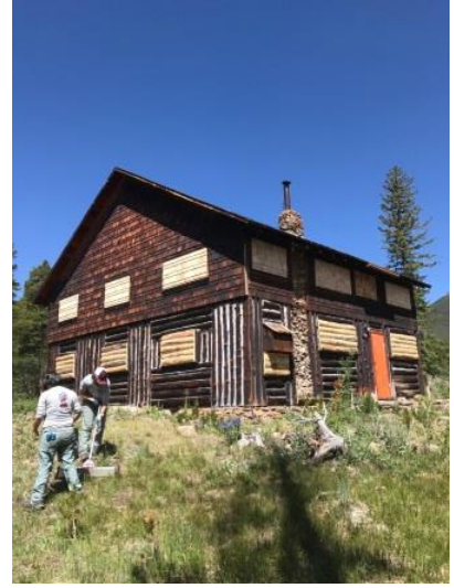
Photo: Completed working to create window coverings to moth-ball the Leiffer Cabin
