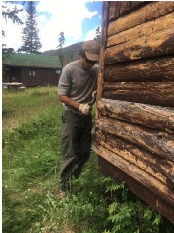
Photo: Crew scraping paint off historic buildings in Green Mountain Village to repaint.
