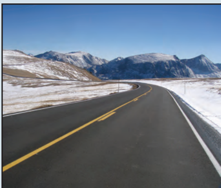
Trail Ridge Road now sports the newly resurfaced look of a well-tended highway. Construction is complete!
