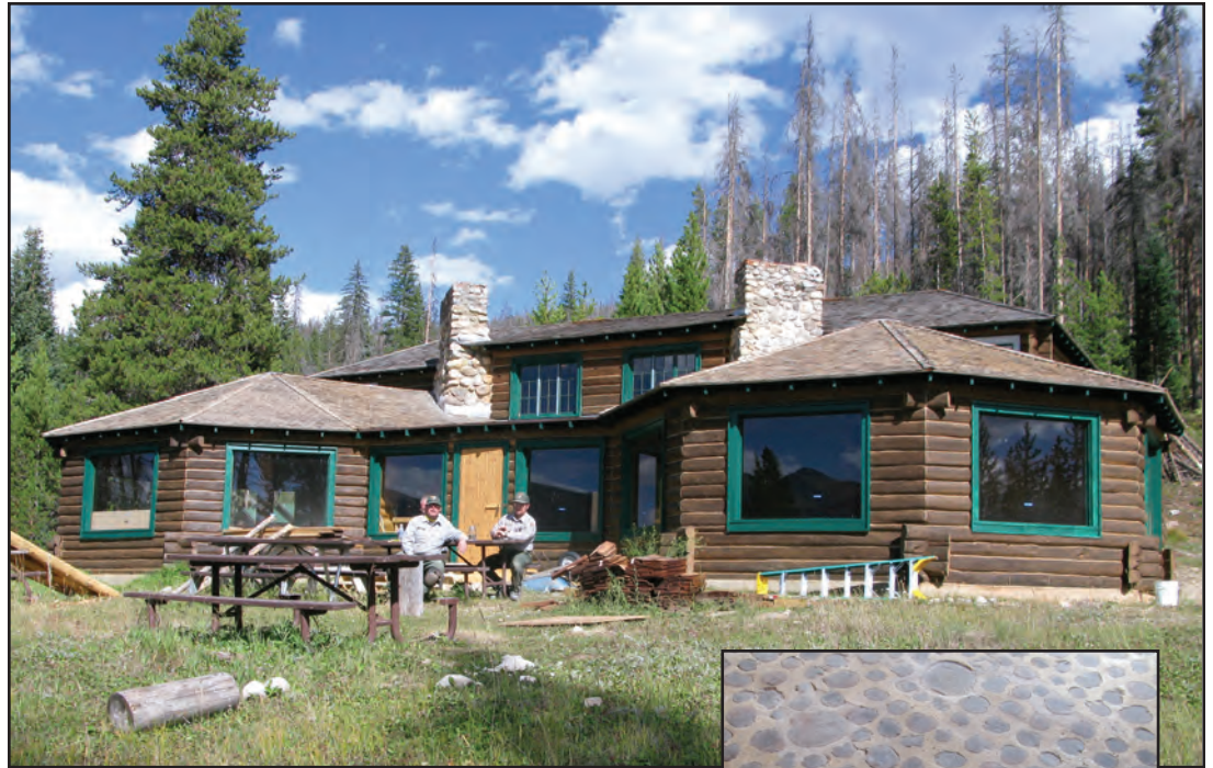
Preservation crew members take a break outside the historic Onahu Lodge last summer as the four-year renovation drew to a close. Not since the renovation of the McGraw Ranch Research Center in 2000 has the crew undertaken such a vast project within the park.
