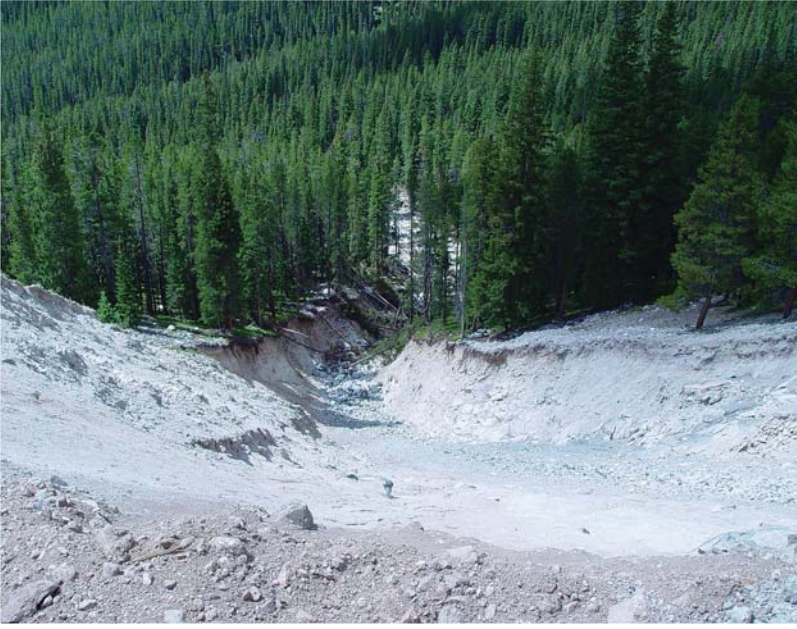
View of the erosion gully directly below the Grand Ditch created by the breach event in 2003. Noted as Zone 1 in Figure 1.
