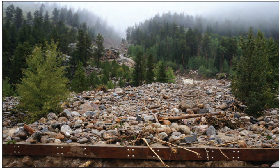
Debris at the Alluvial Fan Bridge following the flood (NPS)
